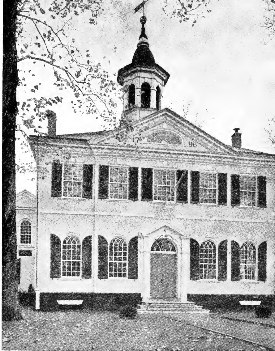
BURLINGTON COUNTY COURTHOUSE, MOUNT HOLLY
